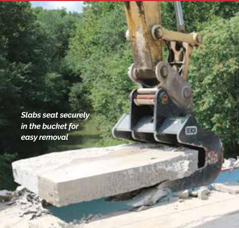
*Slabs seat securely in the bucket for easy removal*
